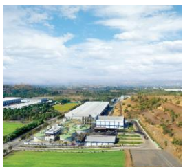
Jain Energy Park Jalgaon (Maharashtra) Solar & BioGas
